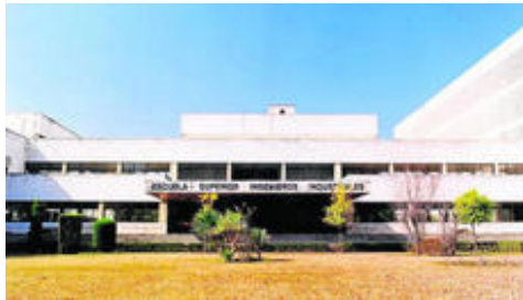
Figure 25. School of Industrial Engineers in Seville in 1975.
